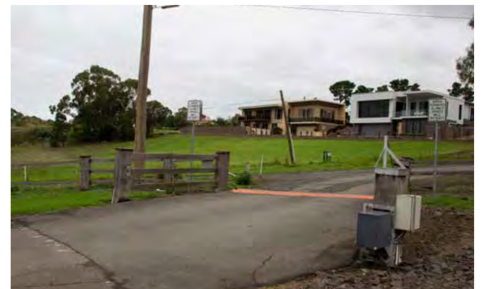
Image 03: View of existing exit gate
