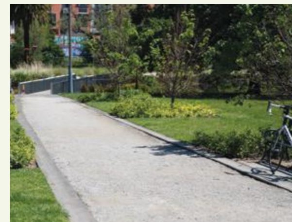
Minimum 3m wide path with unsealed surface and concrete edging to prevent path washout
