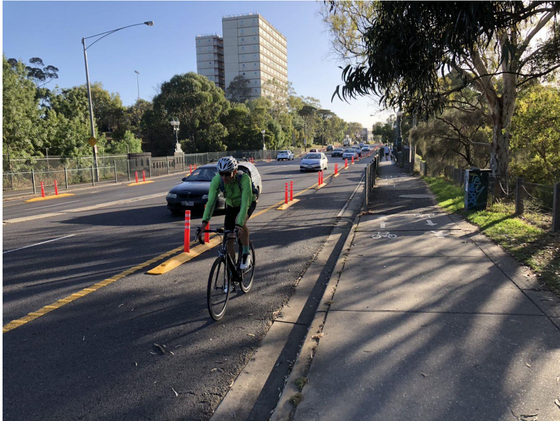
Photo shows the temporary cycling lanes on Heidelberg Rd, Melbourne.
