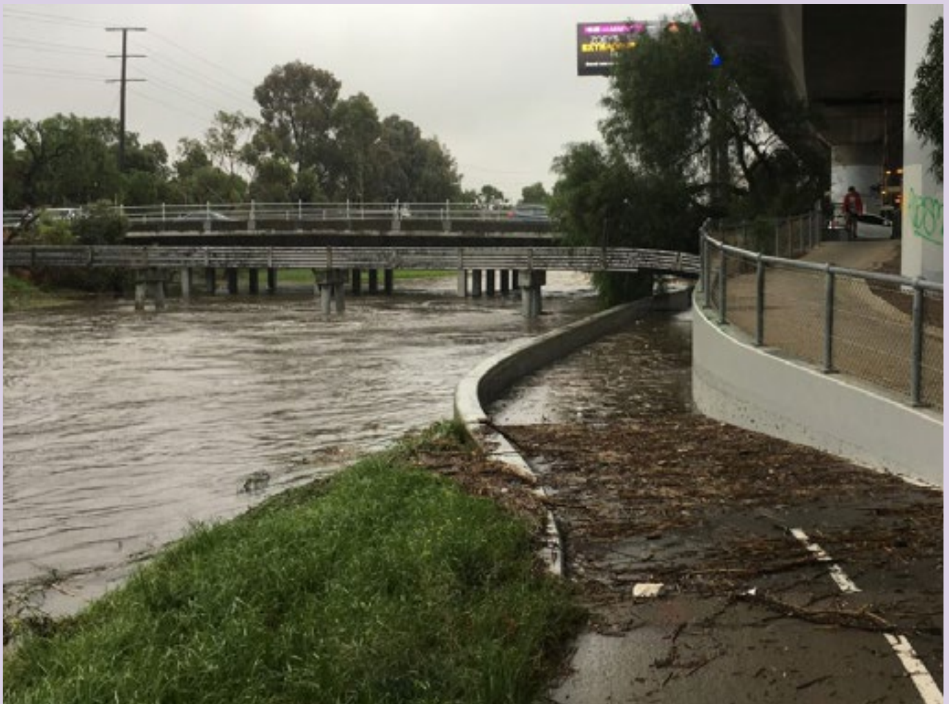
Figure 41 Flooding of the Moonee Ponds Creek at the Macaulay Road Bridge.
