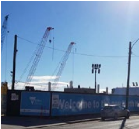
Figure 9 Construction site for the new Arden Station in Arden Central.
