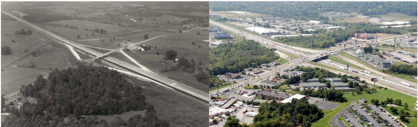
Phase 1 and 2 on Lovell Road and Interstate 75 in Tennessee. Should both major roads be widened yet again as part of phase 3 to “solve” the congestion?
