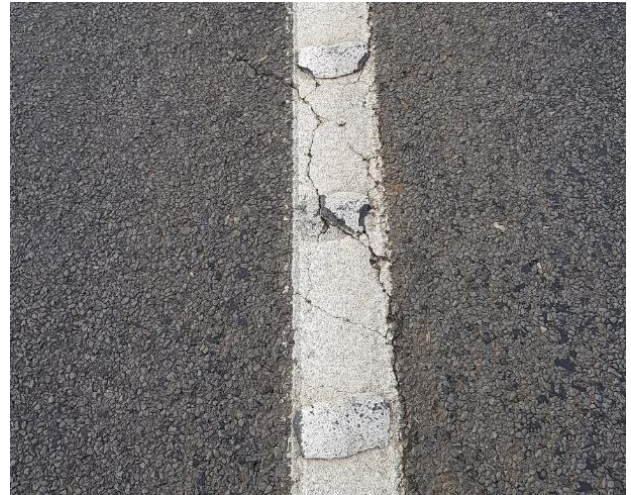
Photo 7.1. Cracking on existing crown
