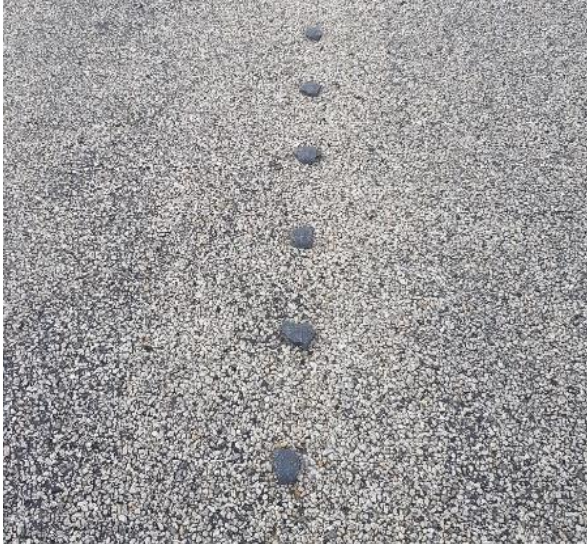
Photo 7.3. Adhesion of audio tactile ribs on older seals
