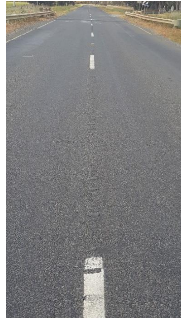
Photo 7.5. Missing audio tactile ribs due to premature failure
