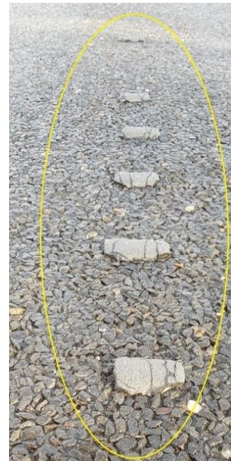
Photo 7.2. Shattering of audio tactile ribs
