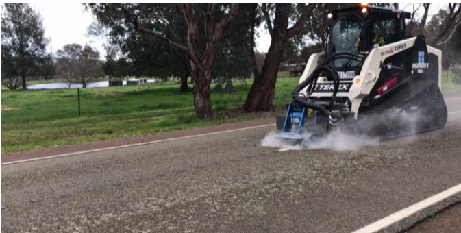
Photo 6.1. Grinding off and removing audio tactile ribs
