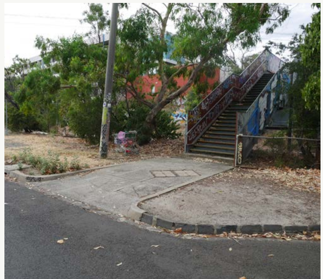
Figure 18: Photo of stairs and bridge over the Sandringham railway line near Elsternwick railway station
