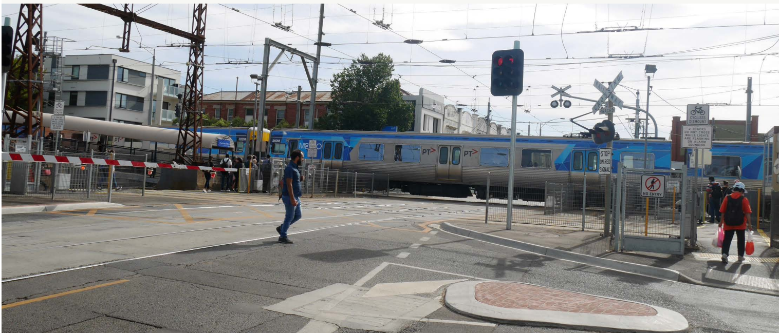
Figure 17: Photo of level crossing outside Glen Huntly railway station
