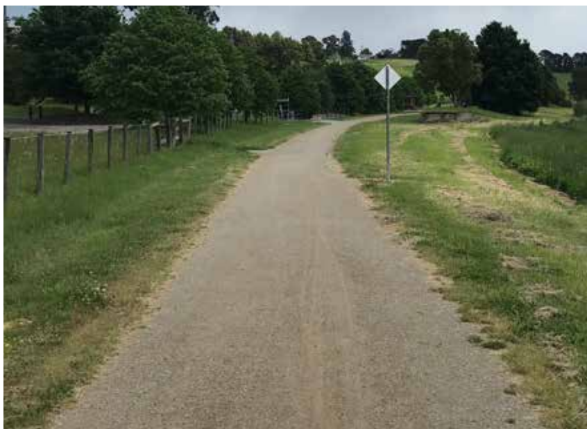
FIGURE 8.1: Regional trail construction material examples. Top: Concrete trail construction (Heathmont Belgrave Trail) Middle: Asphalt surface with concrete strip edging (Anniversary Trail) Bottom: Gravel (Warburton Rail Trail)
