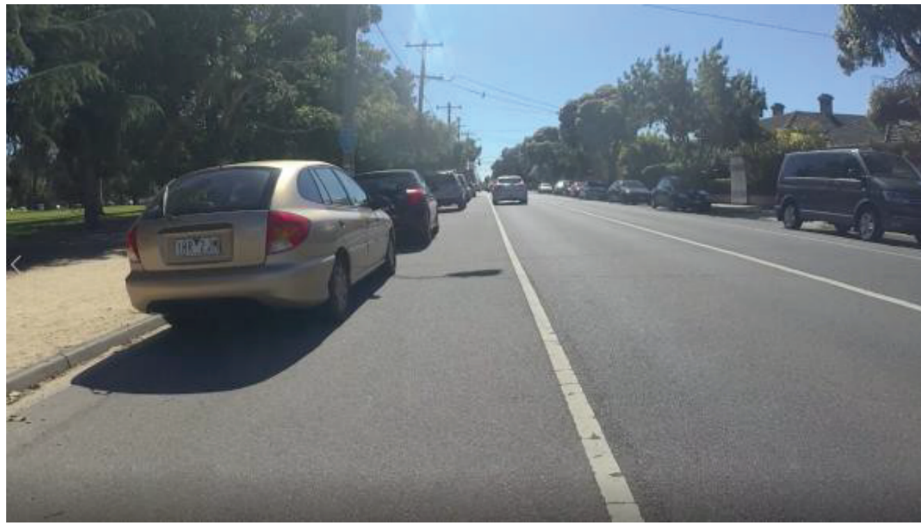
The bicycle lane sits between the traffic lane and parked cars. Cyclists are within the dooring zone for the entire corridor.
