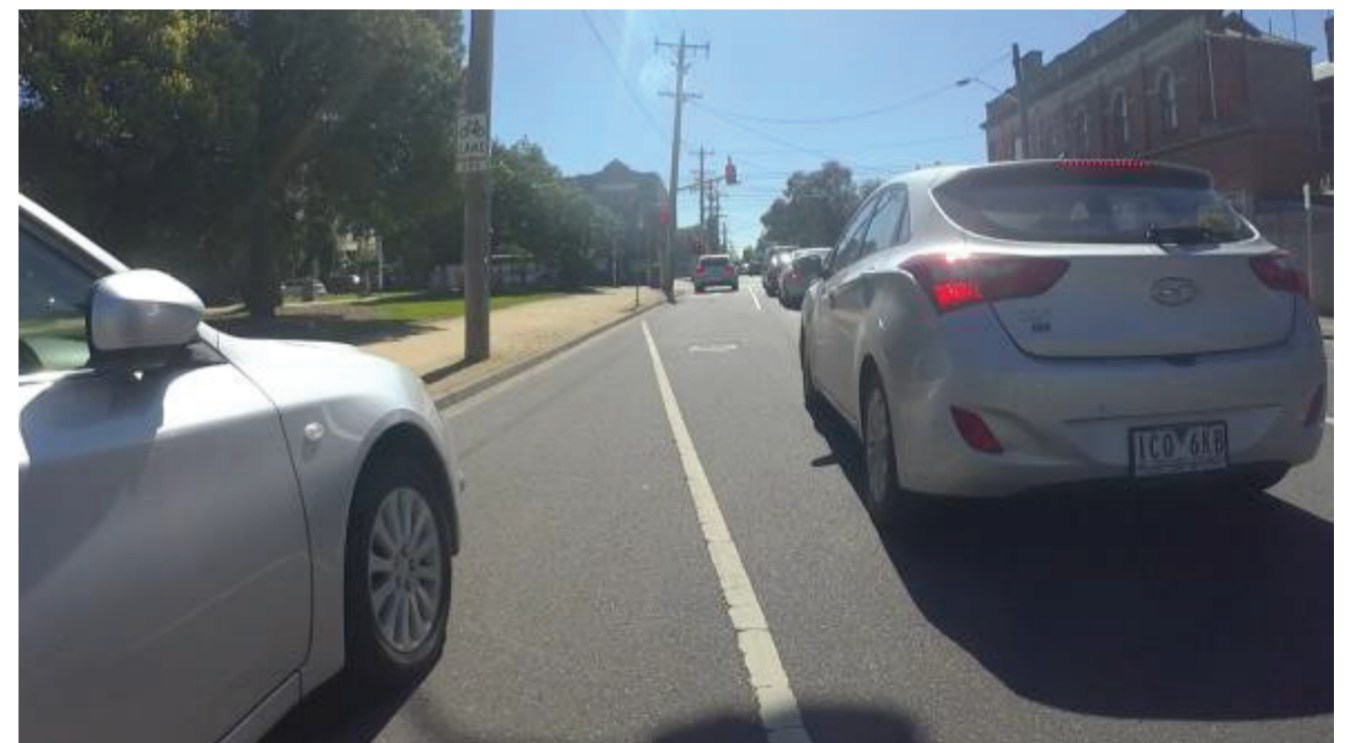
The cycling facilities end at the signalised intersection to make space for two general traffic lanes.
