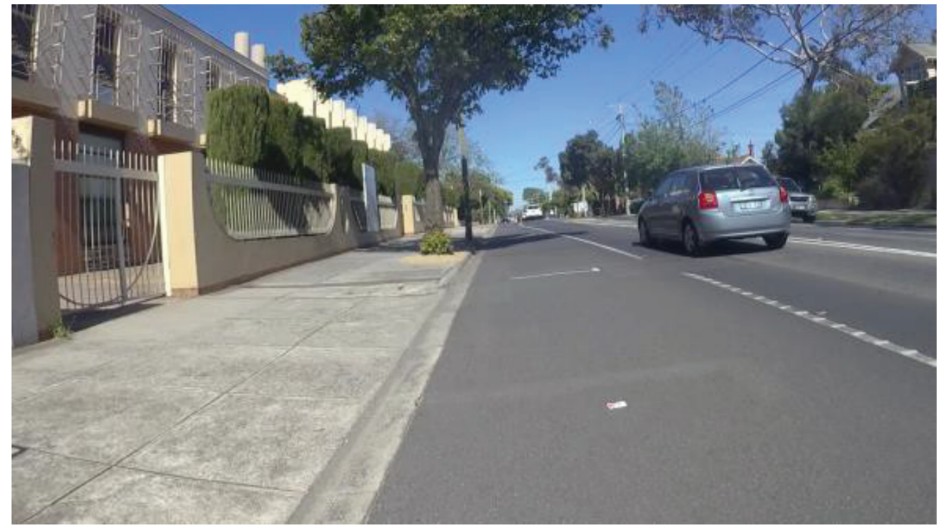
When no cars are parked, the cycling lane is very wide. This could create confusion as to whether it is a trafficable lane for vehicles.
