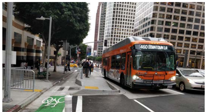
Bus boarding island in Los Angeles, California.
