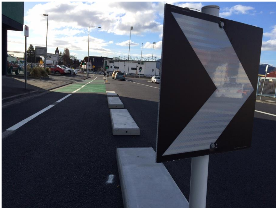
Concrete dividers (Peltro Street, Glenorchy)
