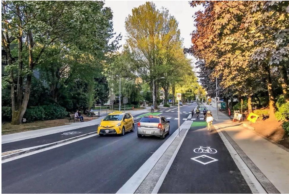
Cycleways raised to footpath level (Vancouver)
