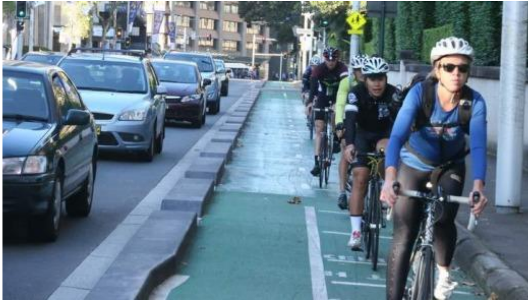
Concrete divider/kerb (Sydney)
