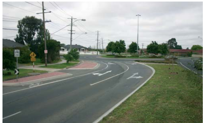
Figure 14 - Two lane, urban roundabout on a busy arterial road in Lalor
