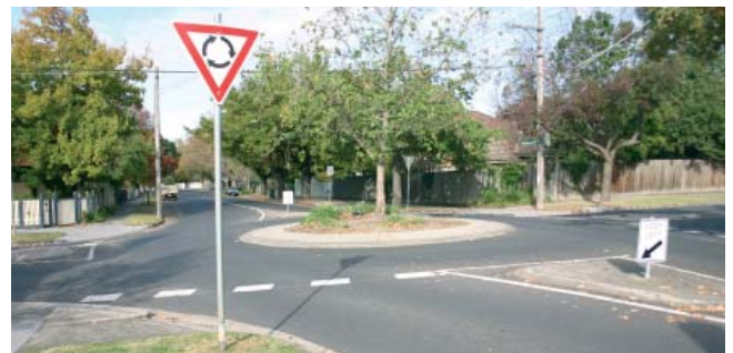
Figure 1 - Single lane roundabout on a local road
