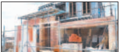
The unfinished Sunshine West house.
