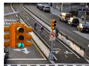
Two-Way Centre Cycle Track, Sands Street, New York (USA) Key difference: physically separated, located in centre of roadway.
