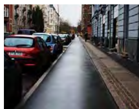
Cycle Track in Toronto (Canada) Key difference: vertical separation and no buffer for door opening.
