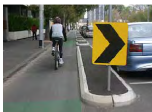
Copenhagen-Style* Bike Lane on Swanston Street, Melbourne Key Difference: Median separation cannot be ridden or driven over. Less space for riders to pass other riders or avoid hazards
