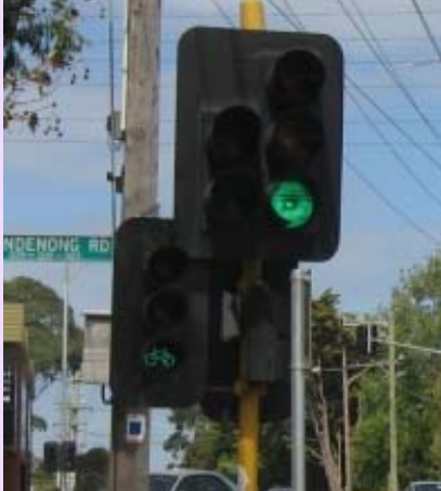
The three aspect cyclist lanterns that have been added to the standard traffic signals for bike riders along Murrumbeena Road at Princes Highway.
