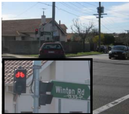
Diagonal bike rider crossing of Malvern Road into Winton Road, Malvern East. During the all red vehicle phase, both the cyclist & pedestrian signals turn green. Note this is likely to be a temporary measure at this location until the parallel bike path is upgraded.
