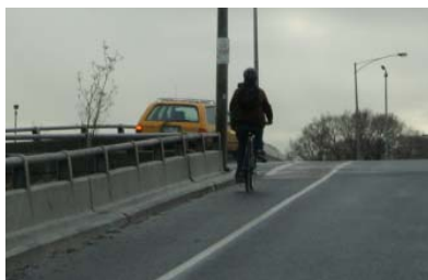
Heidelberg Road bridge over Hoddle Street, where vehicles merging from the left have to cross the bicycle lane
