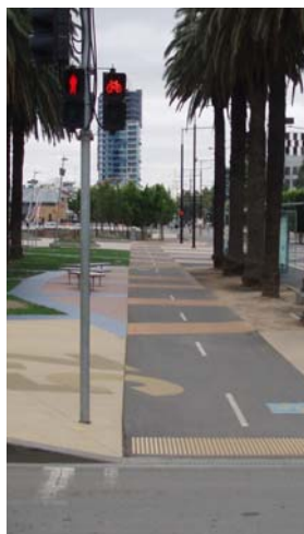
Two aspect cyclist signals run with the pedestrian signal along the shared path through the Docklands
