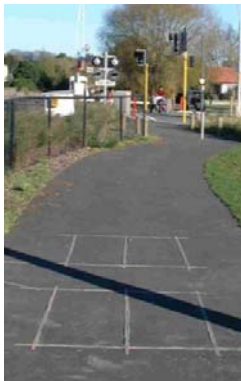
Two sets of inductive loops are used to detect bike riders approaching the signals on the Railway Cycleway in New Zealand.
