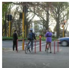
Harper Street crossing in NZ with separate push button detection for bike riders and pedestrians
