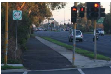
Three aspect cyclist signals run with the vehicle signal at Nepean Hwy/Dendy St, Bentleigh. In this phase no pedestrians were detected and so the 'green man' was not displayed.
