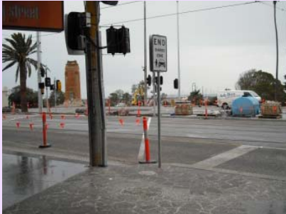
Bike riders and pedestrians have priority at this dwell on red crossing in Fitzroy St, St Kilda
