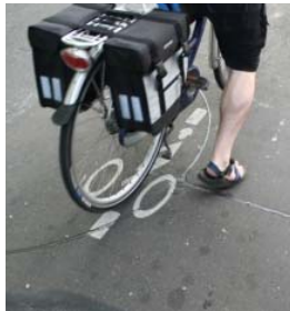
Markings identifying the most sensitive part of an inductive loop in Portland, Oregon (USA)
